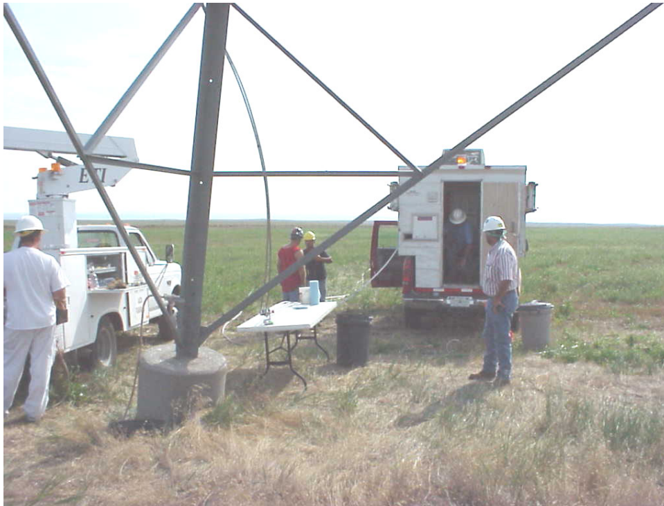
Fig. 1 Maintenance of optical fiber that is inside a ground wire
