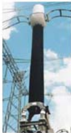
Fig. 2.1: Mounting of HV Current Transformer
