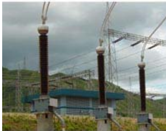
Fig. 2.3: Mounting of HV Coupling Capacitor Voltage Transformer
